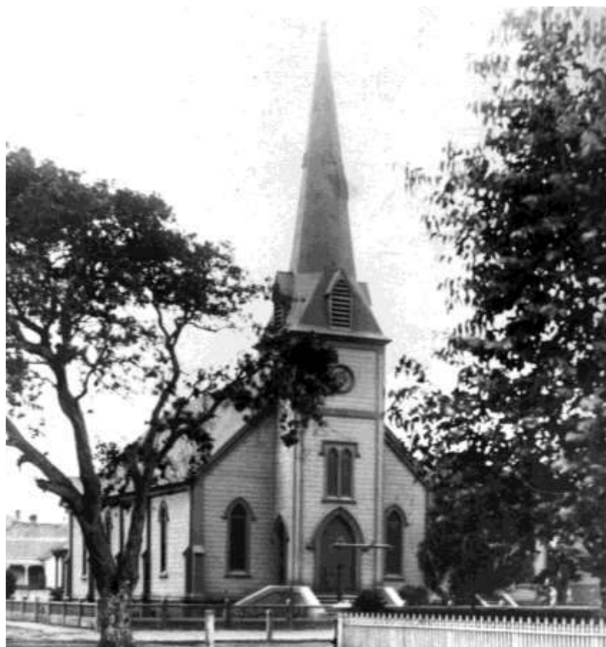
Church building at the corner of Versailles and Central Avenues
